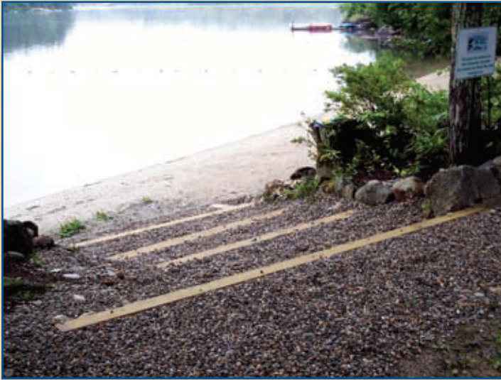
Infiltration steps allow any runoff that reaches the bottom of the hill to sink into the ground before flowing across the beach and the steps provide a safe way for visitors to walk down to the beach.
