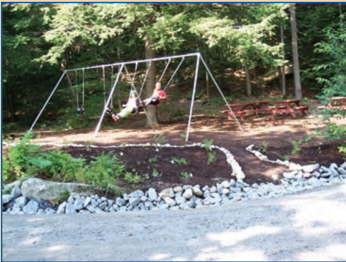
A vegetated buffer and mulch installed on the upper side of the park roadway reduce the amount of water that flows onto the roadway by absorbing water and also help improve the quality of runoff water by soaking up pollutants.
