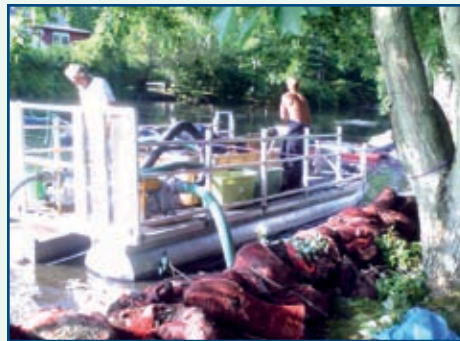
Suction dredging machine at work.
