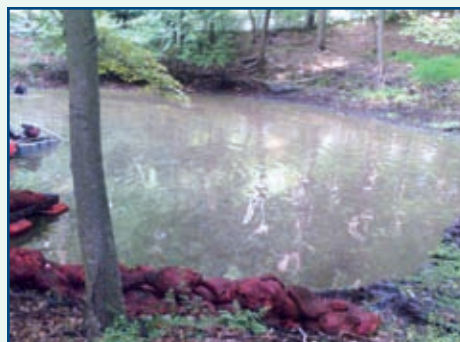
After suction dredging.
