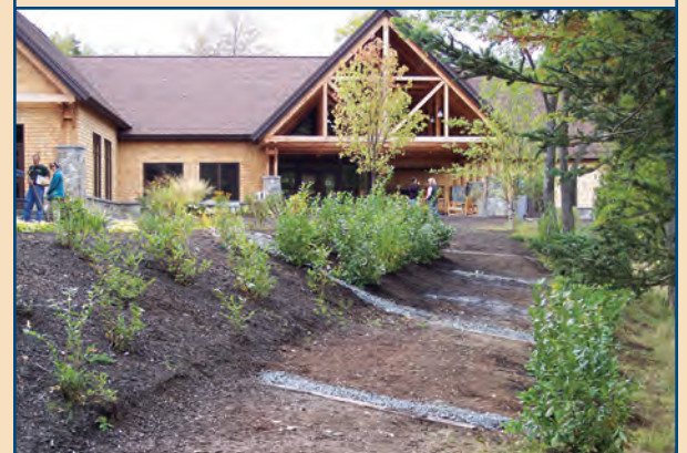
A vegetated buffer and crushed stone water bars were installed at the Eastman Community Association's South Cove Activity Center to reduce the amount of stormwater runoff into Eastman Lake.
