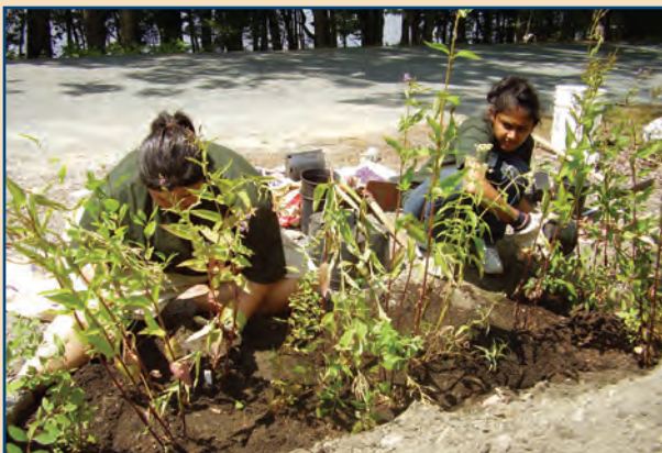
Students planting a rain garden along Goose Pond Road in Canaan.
