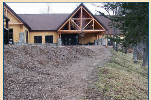
A vegetated buffer and crushed stone water bars were installed at the Eastman Community Association's South Cove Activity Center to reduce the amount of stormwater runoff into Eastman Lake.
