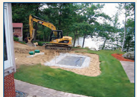
An aerated system like Wastewater Alternatives' The Clean Solution permits a reduced leachfield, often as small as 75 square feet.
