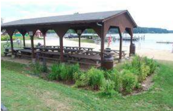
Pavillion after rain garden installation
