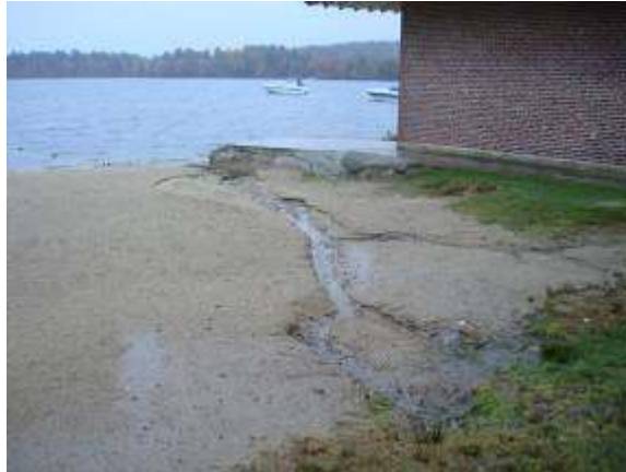
Pavillion drainage before rain garden installation
