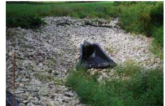
Kelsey Ave outfall with level spreader
