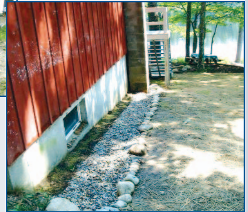
Right: A dripline trench was installed to catch water that runs off the roof allowing it to sink into soil below instead of running downhill and picking up pollutants before flowing into the lake.
