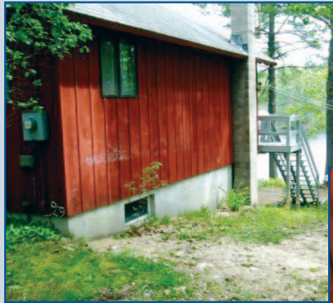
Right: A dripline trench was installed to catch water that runs off the roof allowing it to sink into soil below instead of running downhill and picking up pollutants before flowing into the lake.
